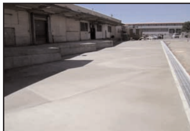
Dock work with Kares Construction
